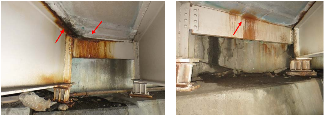
Figure ES7: Typical Slab Delamination at Bridge Ends
