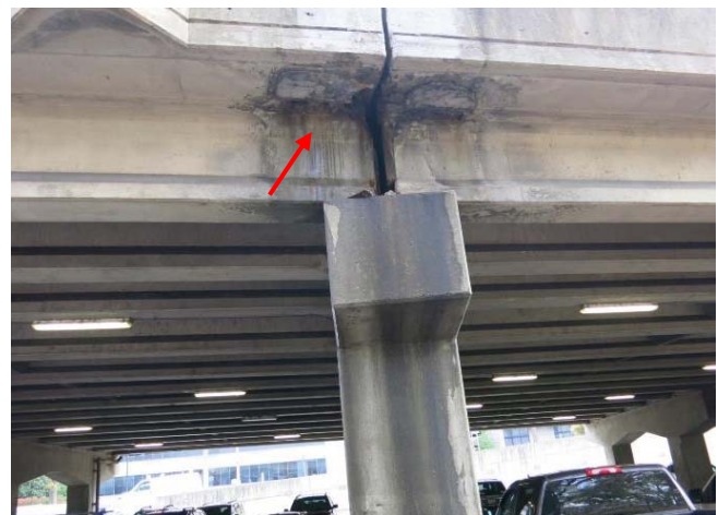
Figure ES5: Typical Pier Joint Leakage and Concrete Damage
