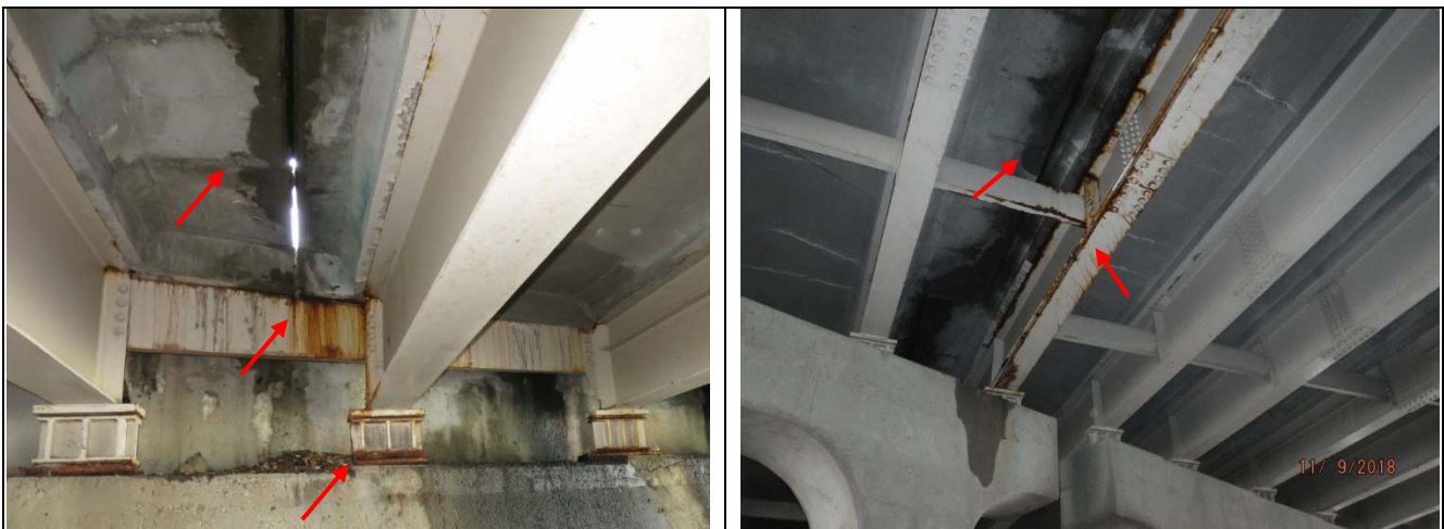
Figure ES8: Typical Median Joint Leakage and Corrosion
