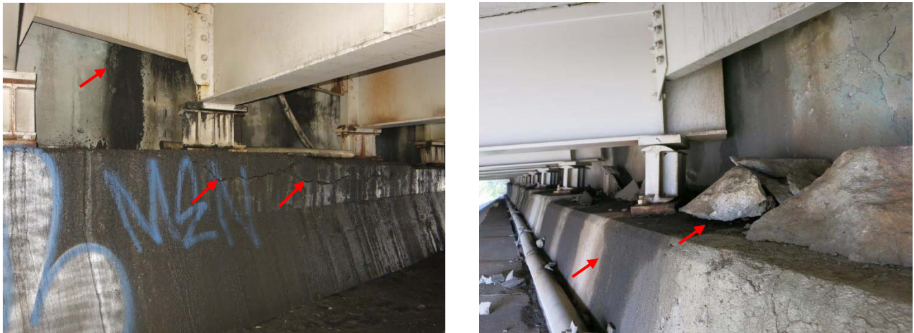
Figure ES3: Typical Abutment Joint Leakage and Concrete Damage
