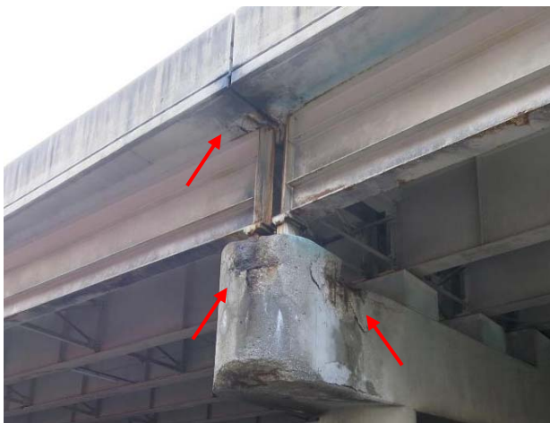
Figure ES5: Typical Pier Joint Leakage and Concrete Damage
